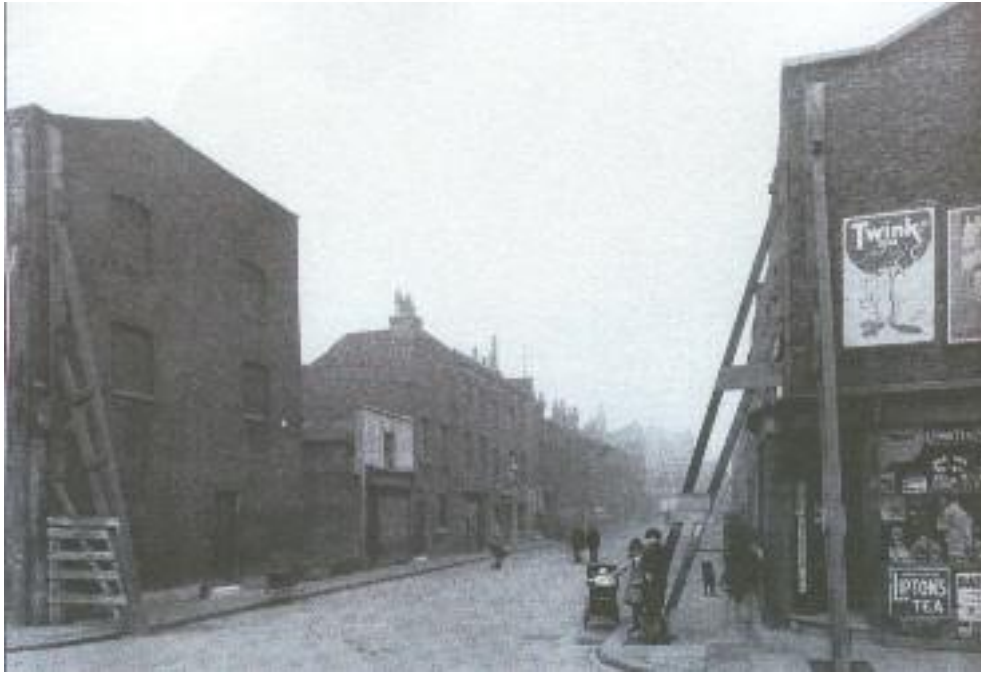
Corner of Esher St and Vincent St
