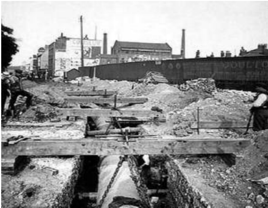
Gas pipe laying in Battersea
